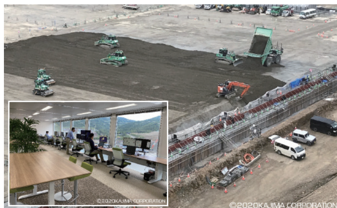
A 4 CSEL at work (@CSG Dam 2020)
